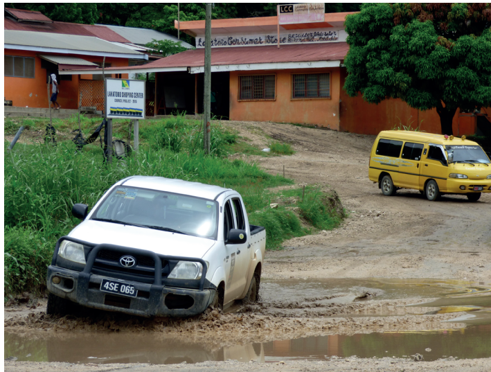
Figure 6. A typical wash out after heavy rainfall. Lakatoro, Vanuatu, 2017 (Photo credit: Ana Terry).
