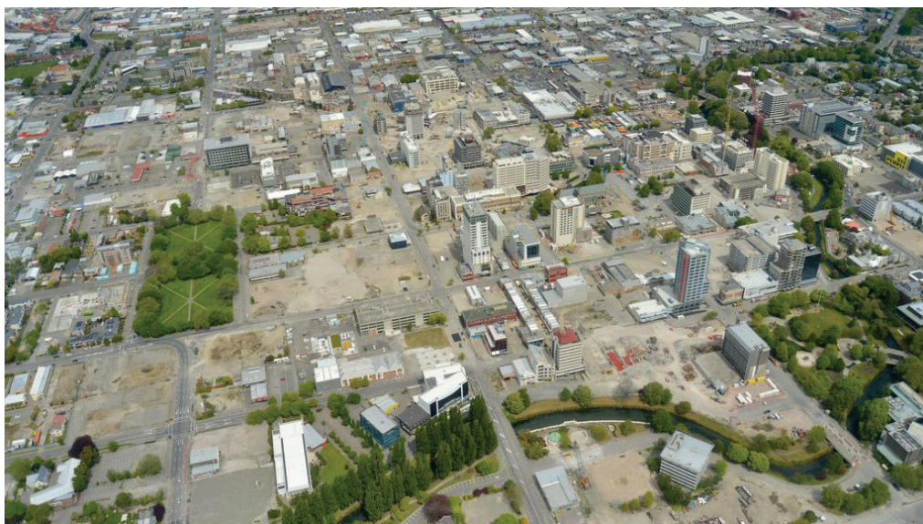
Figure 1. An aerial photo showing the extent of Christchurch's Central Business District cleanout since 22 February 2011 Christchurch Earthquake (Image: Copyright Chris Hutching, 2012. Reproduced with permission).
