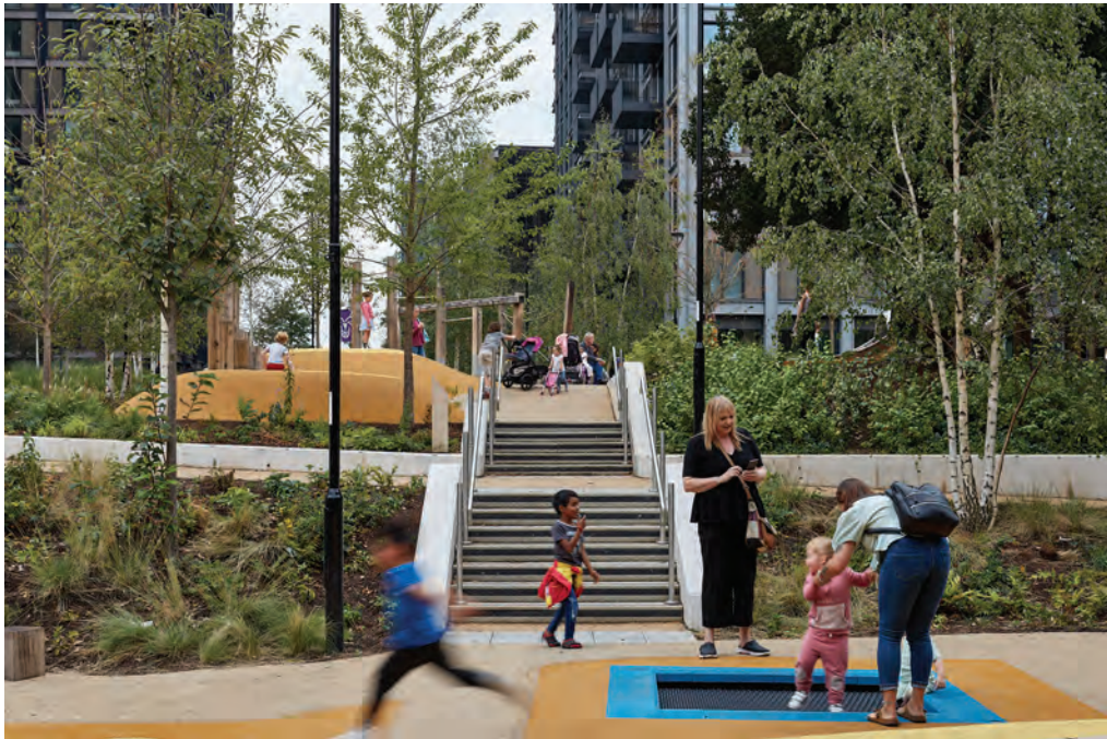
Figure 3. Queen's Quarter is a high-density residential scheme of three towers nested within an intensively landscaped ground play, incorporating an array of play spaces for all ages.
