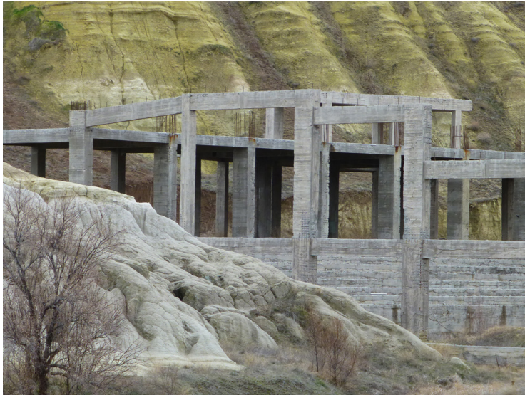
Figure 4. Abandoned construction. Cappadocia, Turkey. Photograph: Ross T Smith, 2015.
