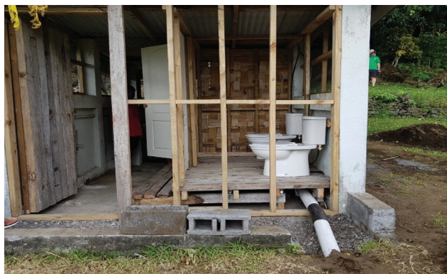
Figure 4. Shower and toilet block nearing the final stages. Source: Authors.
