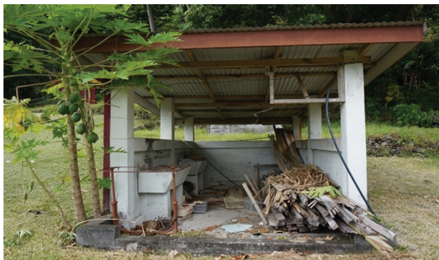
Figure 3. Existing structure chosen for conversion to a toilet and shower block. Source: Authors.
