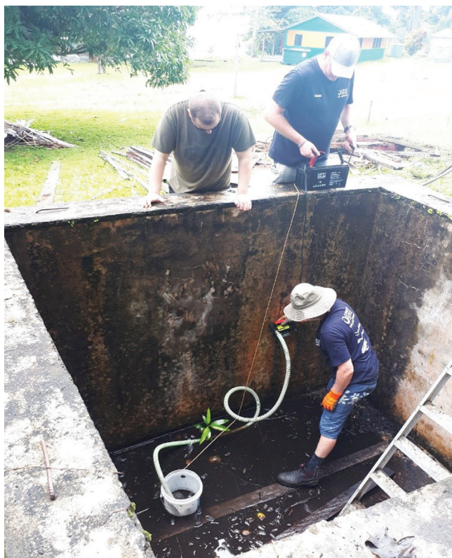
Figure 7. Rehabilitation of existing ground water tanks. Source: Authors.
