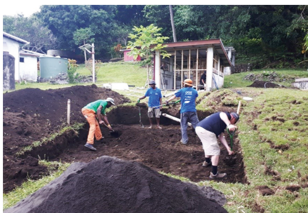
Figure 5. Construction of sanitation field for renovated toilet and shower block. Source: Authors.
