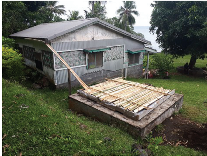
Figure 8. Bamboo covers and guttering were provided for existing underground tanks. Source: Authors.
