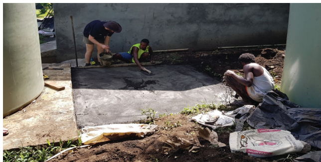
Figure 6. Cement base construction for a new community water tank. Source: Authors.
