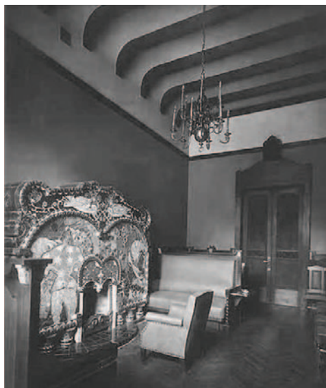
Figure 9. Novikov apartment house, 11 Kolokol'naia Street, St Petersburg.
